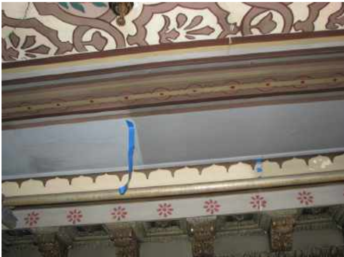
ABOVE The images are all from the Council Chamber ceiling. Cleaning with plain water was quite effective and considered to be more than adequate. Only gentle scrubbing action was required to dislodge the dirt. No paint loss was observed.
