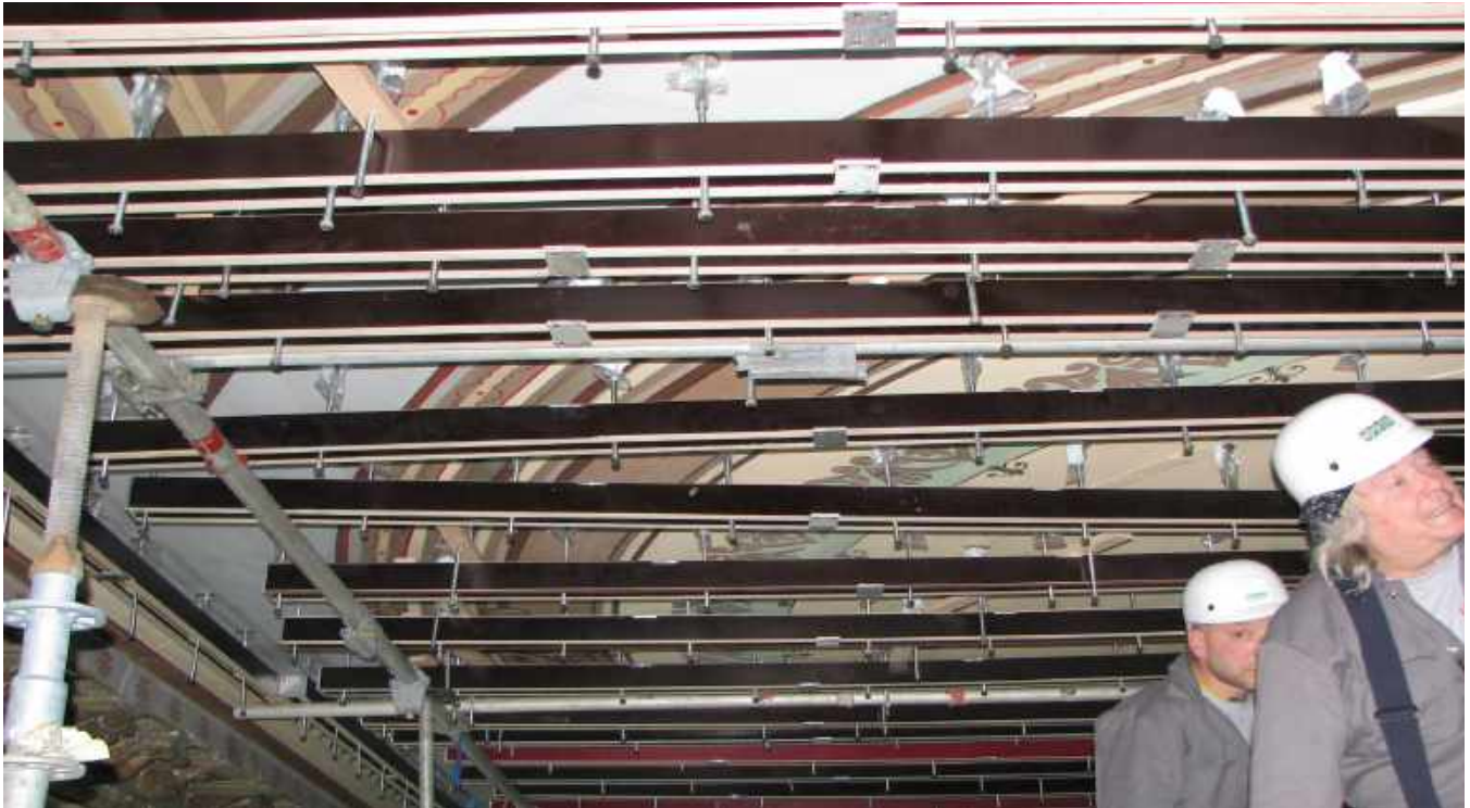
ABOVE and BELOW Before the attic could be safely cleaned, a system of plaster support beams was put in place to carry the weight of the plaster. 260 beams were used, each providing up to 12 individually adjustable support points. The ceiling surface was protected by a soft foam pad attached to the contact point. Because the system offers great flexibility, the individual contact points could be selected on the basis of providing support and not damaging any “freehand” Pindikowski painting.
