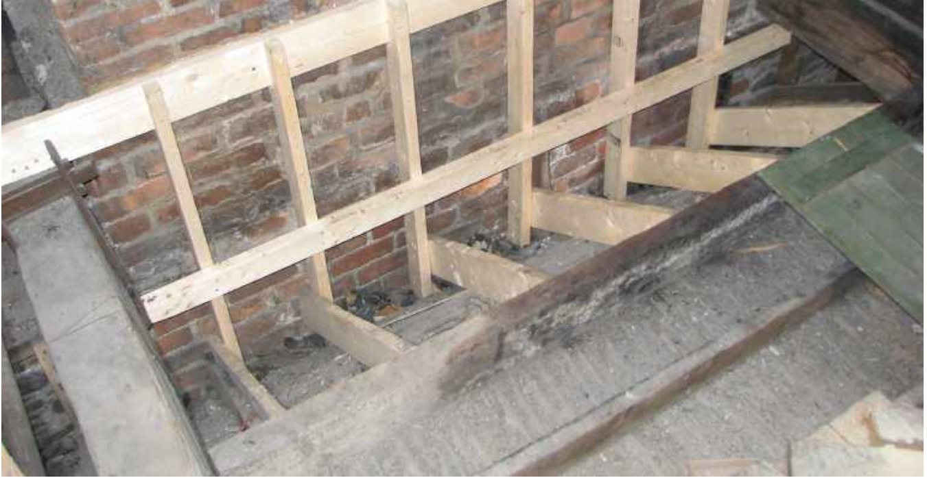
ABOVE New framing was provided to support the cornice against the chimney of the Council Chamber. This had never been repaired after the 1939 fire.
