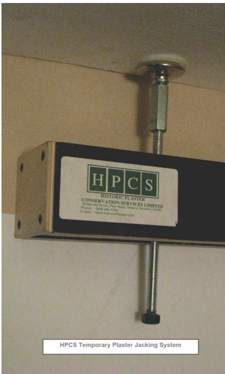
ABOVE and BELOW Before the attic could be safely cleaned, a system of plaster support beams was put in place to carry the weight of the plaster. 260 beams were used, each providing up to 12 individually adjustable support points. The ceiling surface was protected by a soft foam pad attached to the contact point. Because the system offers great flexibility, the individual contact points could be selected on the basis of providing support and not damaging any “freehand” Pindikowski painting.
