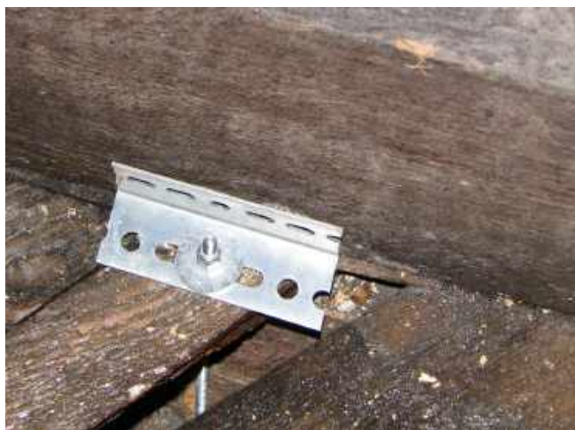
In the attic above the medallions, the new anchors terminate with large washers, a section of perforated angle and a non-slip nylon lock nut.
