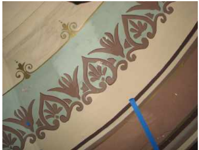
ABOVE The images are all from the Council Chamber ceiling. Cleaning with plain water was quite effective and considered to be more than adequate. Only gentle scrubbing action was required to dislodge the dirt. No paint loss was observed.
