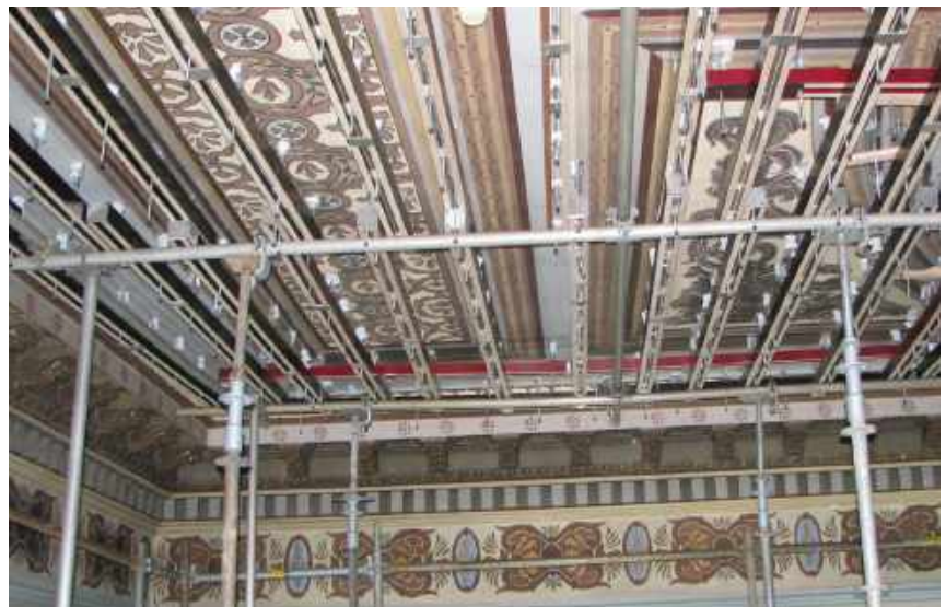
ABOVE The HPCS Temporary Plaster Jacking System requires the installation of a conventional “System Scaffold” working level deck. The structure of the scaffolding system is further used to erect a rigid and adjustable superstructure just below the flat surface of the decorated ceiling.
