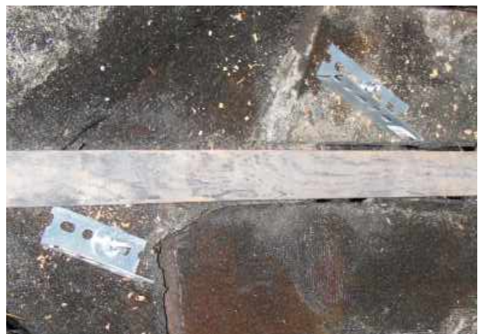
In the attic above the medallions, the new anchors terminate with large washers, a section of perforated angle and a non-slip nylon lock nut.
