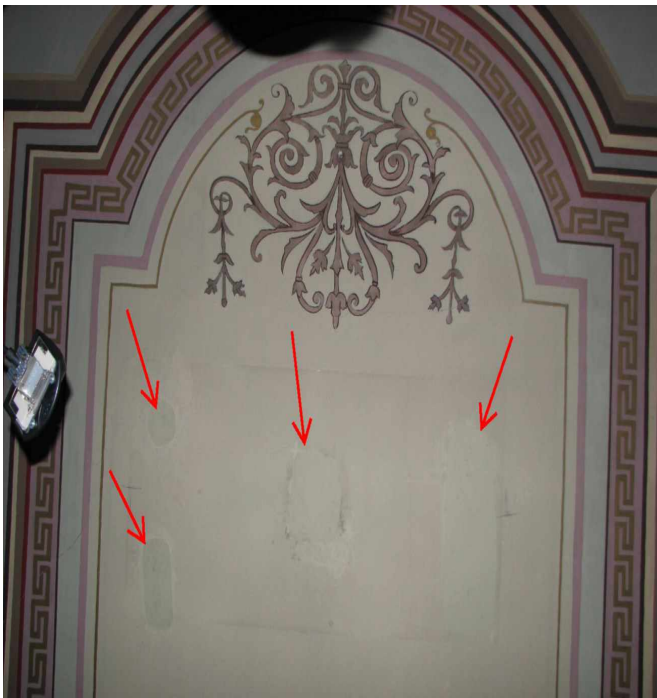
Holes in the soffit had previously been patched with adhesive paper and printed to more or less match the ceiling.
