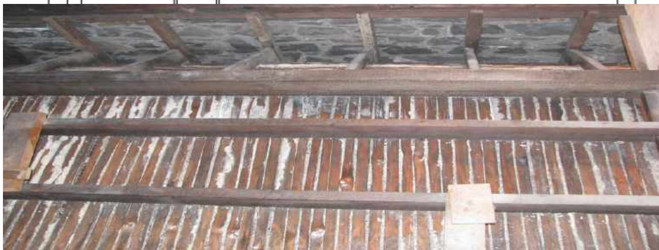
ABOVE Illustrates a section of ceiling that is cleaned and ready for consolidation treatment.
