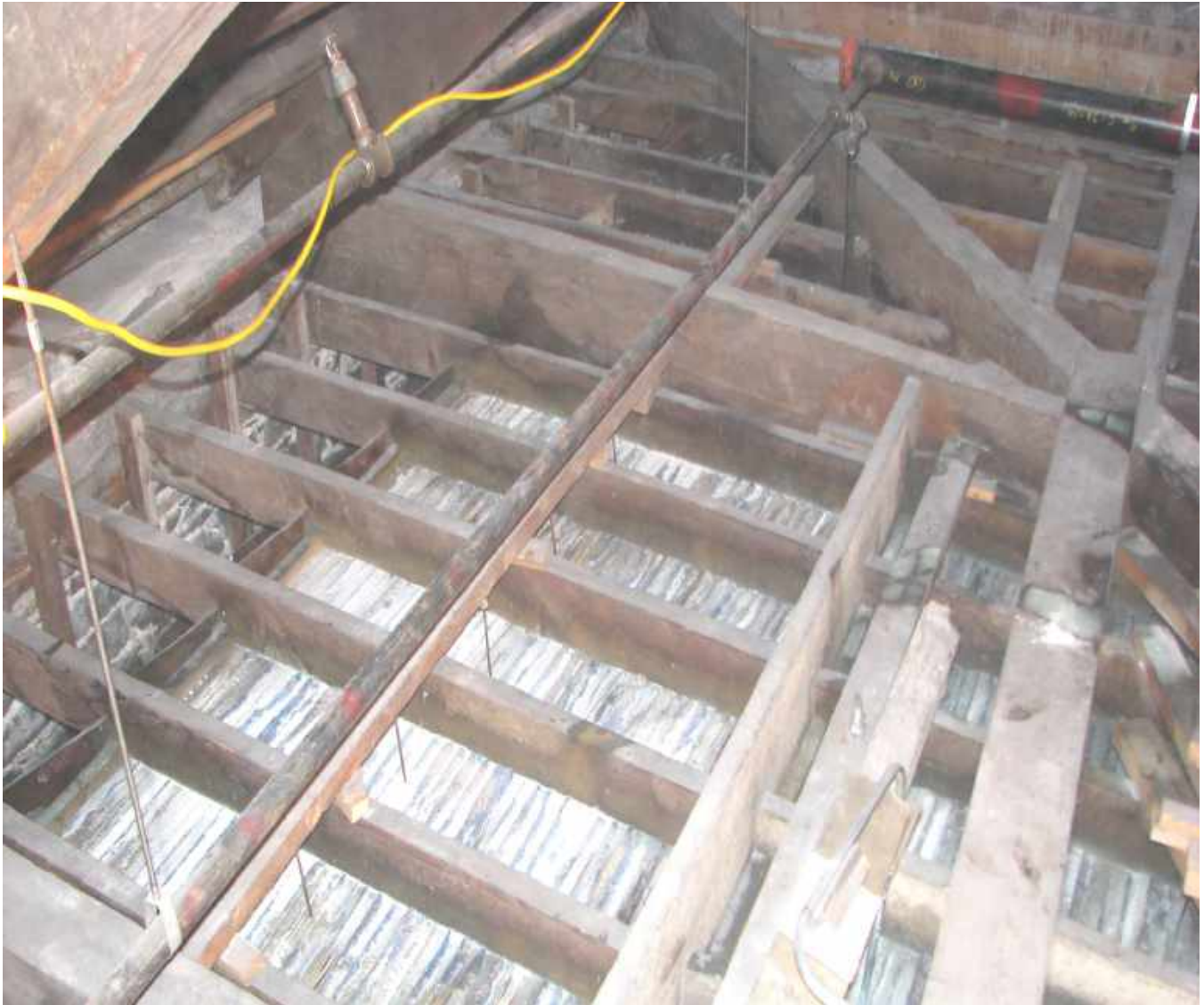
ABOVE Section of ceiling after spray application.
