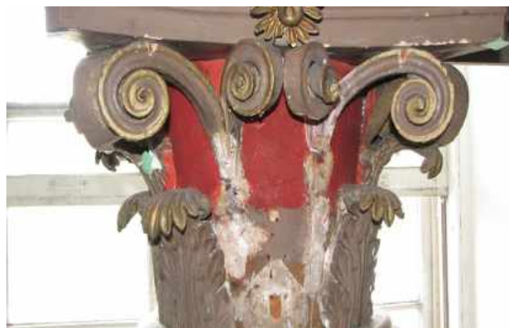
ABOVE Capitals and other ornament below the galleries were in particularly distressed condition.
