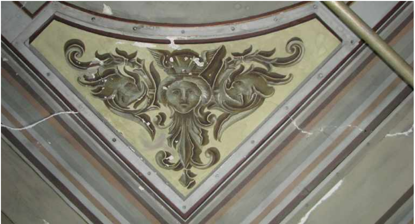
ABOVE The Murphy frame in this case is made to follow the perimeter of the Pindikowski painting.
