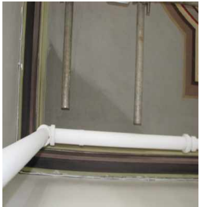
Triangular section (southeast corner) of CC ceiling left uncleaned for client review.
