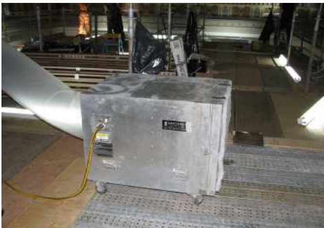
ABOVE The 2500 c. f. m. “Negative Air” unit equipped with Hepa filters was constantly used to clean the air in the project work area.
