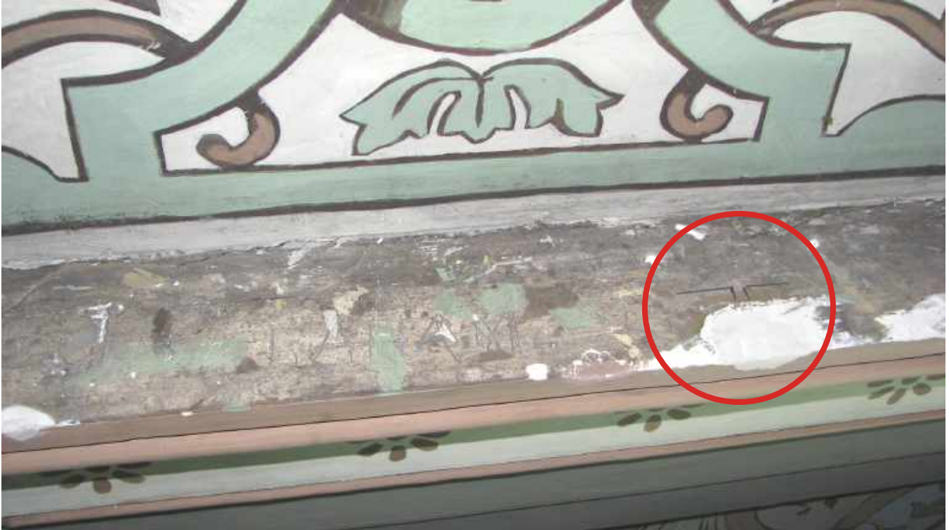
ABOVE J. Graham signed by carving beside a set of stencil layout marks seen in the circle.
