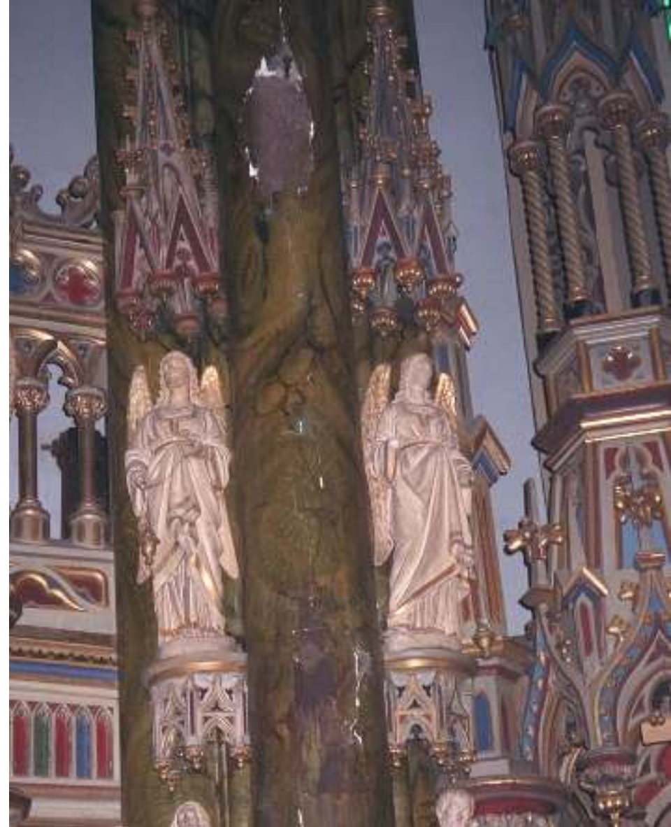
Faux marble finish on plaster columns
