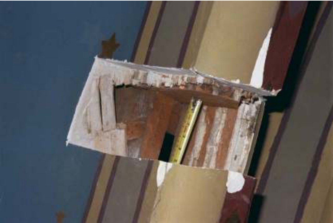
A RIB CUT OPEN FOR INVESTIGATION
