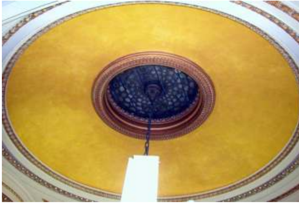
The finished upper dome.
