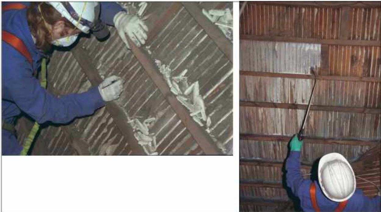
Figure 3: Left: Technician Testing Keys and Right: Technician Applying Dilute Resin
