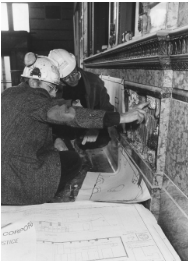
Figure 6. Once the test indicated that the procedure located the plaster adhesive patches with 90% accuracy, the survey continued.
