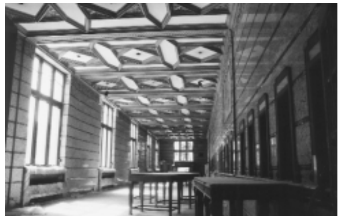
Figure 2. Postal hall of the Dominion Public Building is clad floor-to-ceiling in marble.
