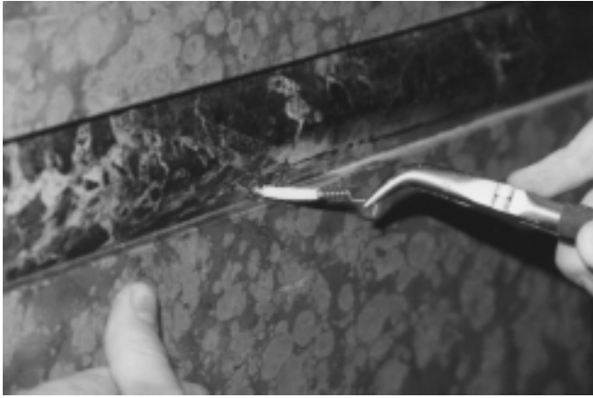
Figure 11. Stainless helical spring is inserted. Note the tail is formed to fit the hole being drilled in Figure 9.
